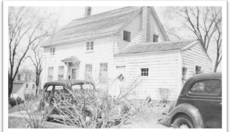
133 North Street, 1940's
